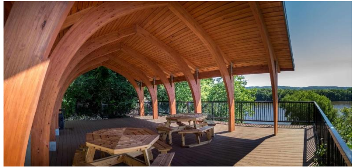
Figure 22: Marquette-Joliet Bridge Scenic Overlook
